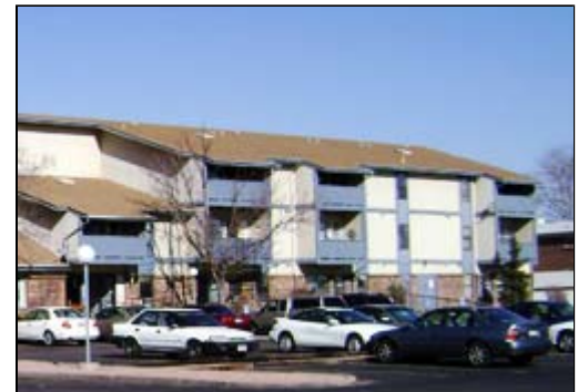
TCAP funding will make improvements to Denver Gardens in southeast Denver, CO, possible.
