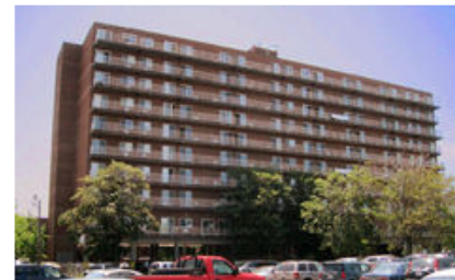
Heritage Apts. in Malden, MA, will undergo a substantial rehabilitation. Heritage is one apartment complex included in WNC Institutional Tax Credit Fund 34, L.P.
