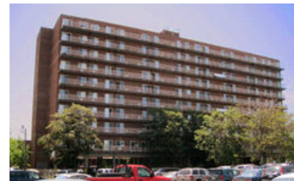
Heritage Apts. in Malden, MA, will undergo a substantial rehabilitation. Heritage is one apartment complex included in WNC Institutional Tax Credit Fund 34, L.P
